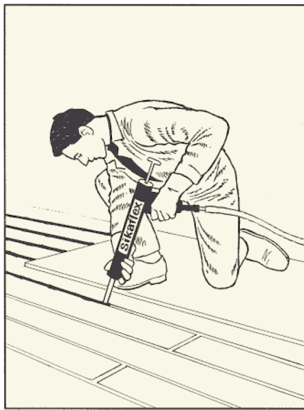
Deck caulking procedures
